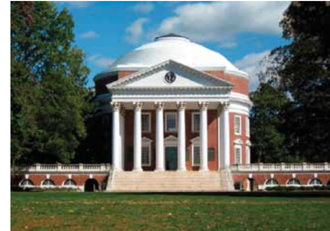
Rotunda (1822) University of Virginia, Charlottesville, Virginia.
