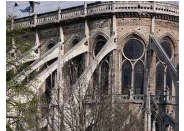
Flying buttresses, exterior of Notre-Dame.
