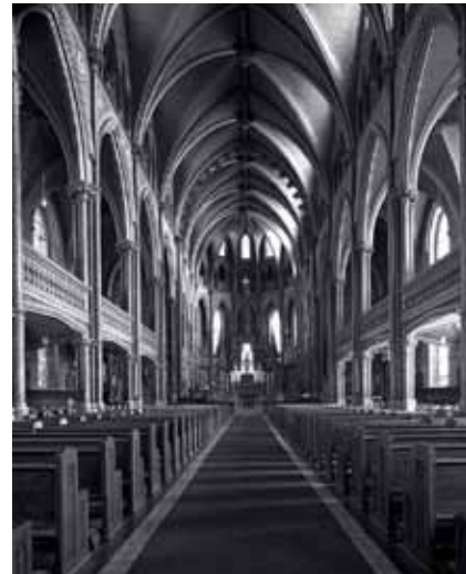
Interior with ribbed vaults in the nave of Notre-Dame.
